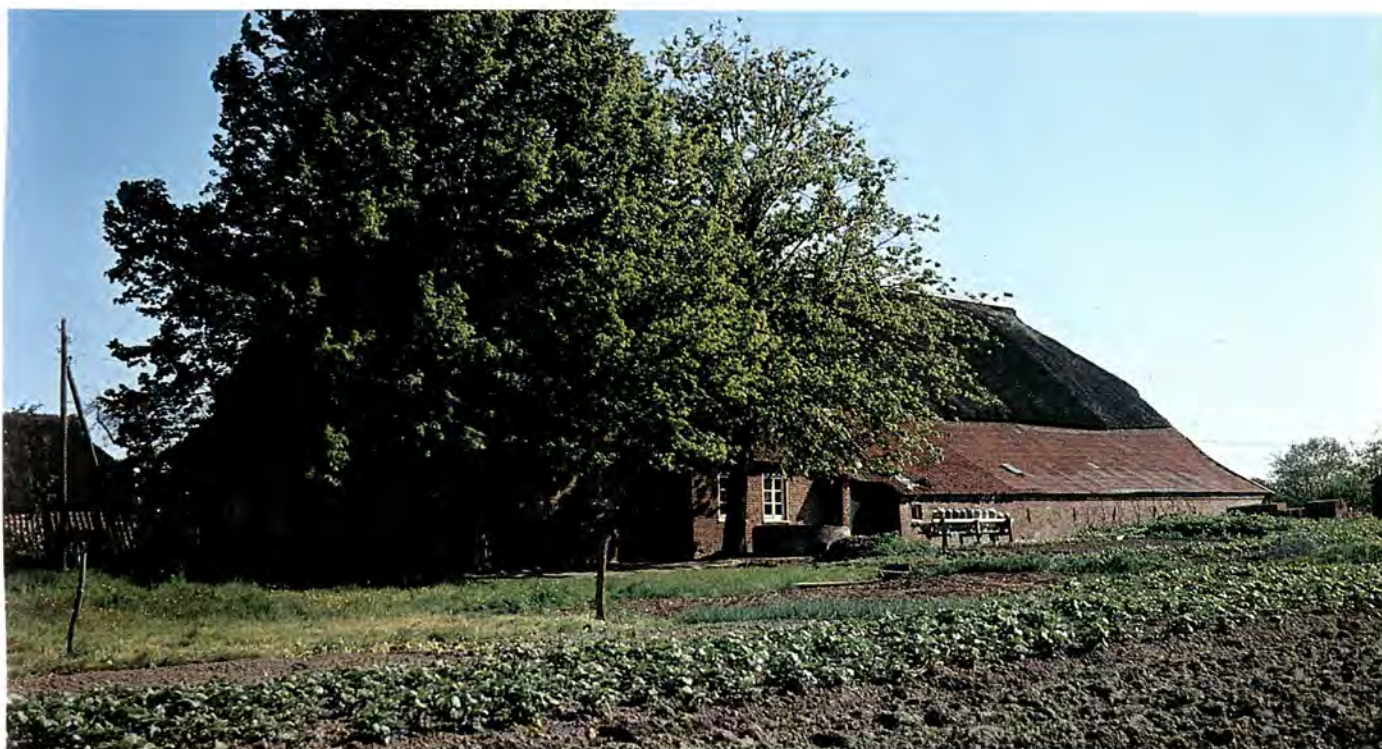
View of the farmhouse, erected in 1864, where the hoard was found during modernisation work; view from the fields.
